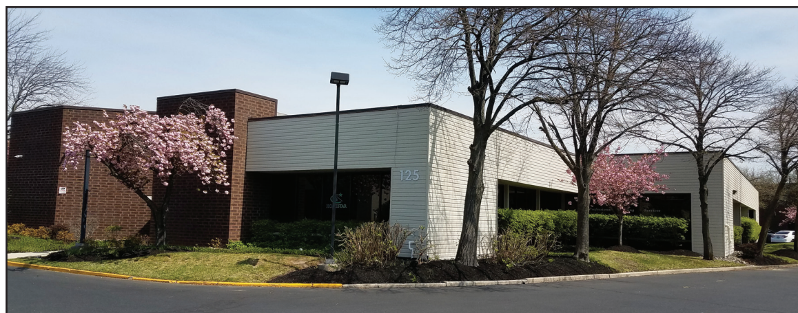
East Gate Business Center
